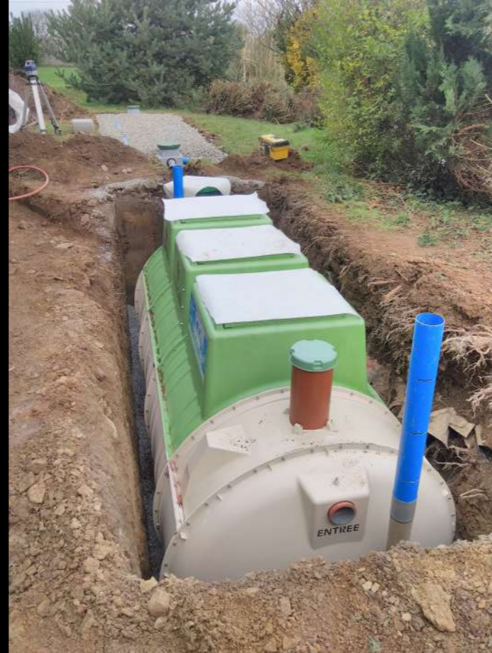
Tricel Seta being installed
